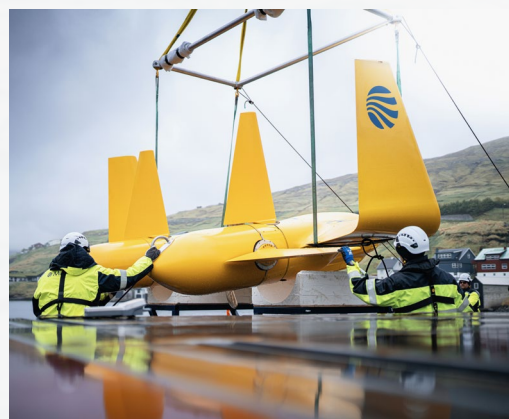
The first "Dragon 4" power plant unit being lifted into the sea in Vestmanna, Faroe Islands.
